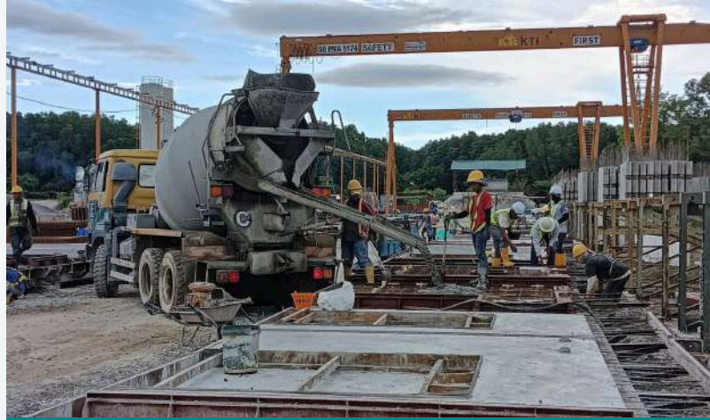
Figure 4: Precast Casting Yard near Project Area at Kota Kinabalu, Sabah
