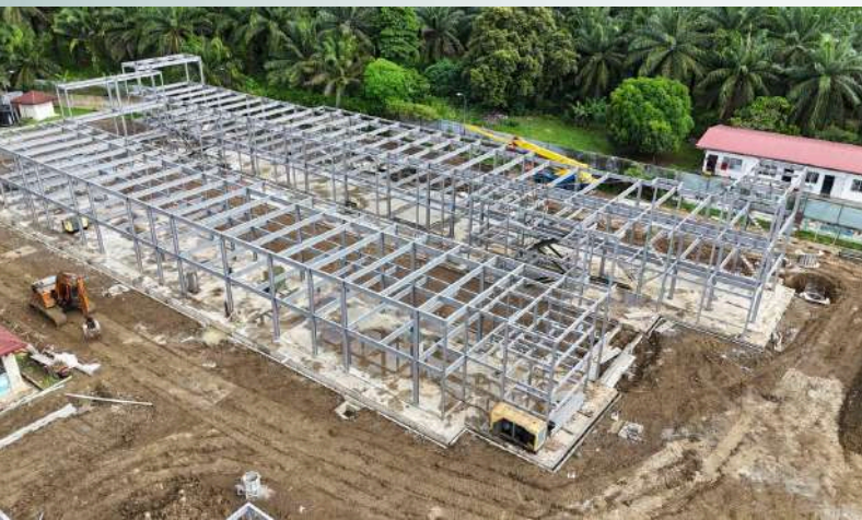
Figure 3: IBS project using steel framing – Sekolah Kebangsaan Tagasan at Semporna
