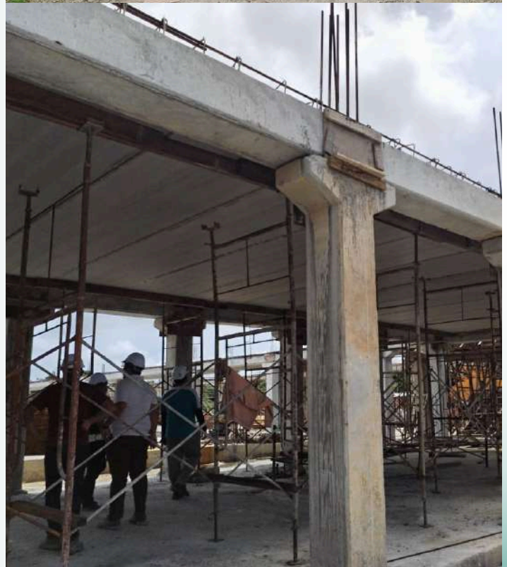
Figure 1: Site Visit on IBS Project in Sarawak
